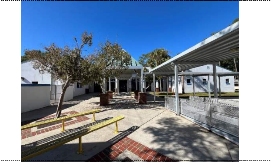
Photo 56 - Entrance to building 3.
